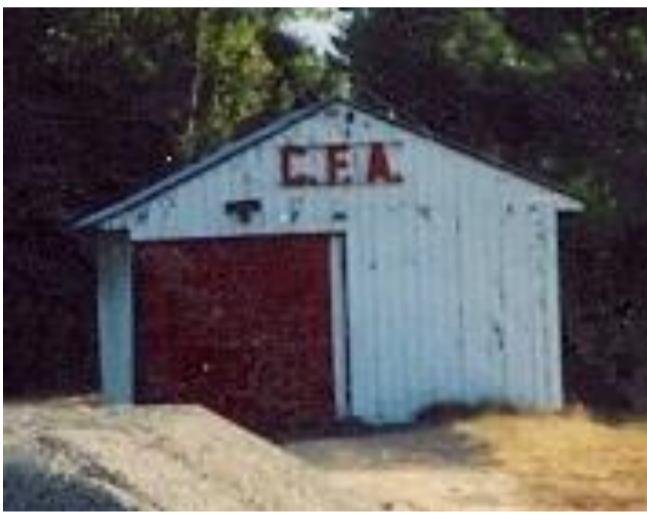
Buxton's first fire shed, under construction (top right), and completed (left). The C.F.A. lettering can still be seen in our current Engine Bay in 2024.
